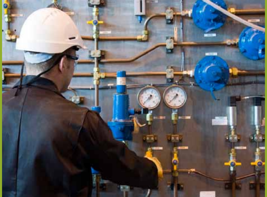
The Hot Isostatic Press (HIP) rig at Workington Laboratory. NNL has been working with the Australian Nuclear Science and Technology Organisation (ANSTO) to develop a process for the treatment of plutonium residues. Using the HIP process produces a stable ceramic matrix suitable for long-term storage
